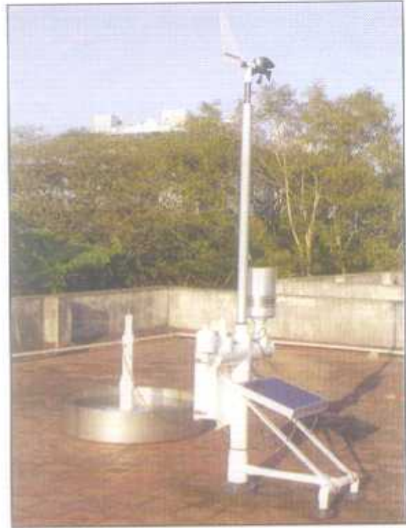
Automated Solar Powered Weather Station (NEERI)
