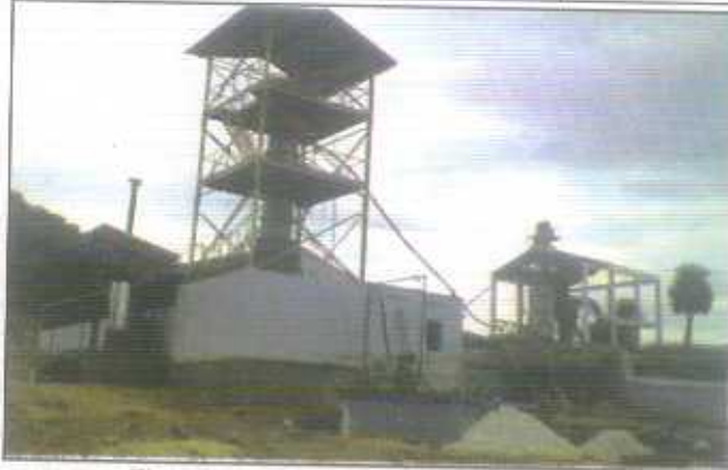
Flotation column under installation at M/s. Calpro Mineral Technologies Pvt. Ltd., Salem, Based on NML technology
